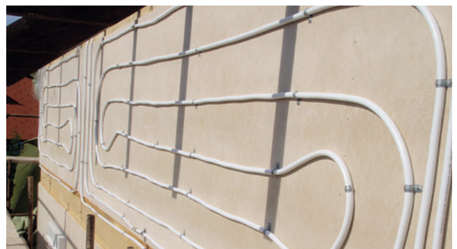
2 Active thermal barrier against heat
