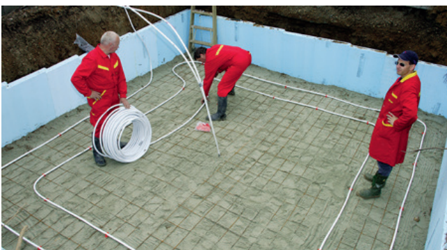
1 Underground cold exchanger in ground
